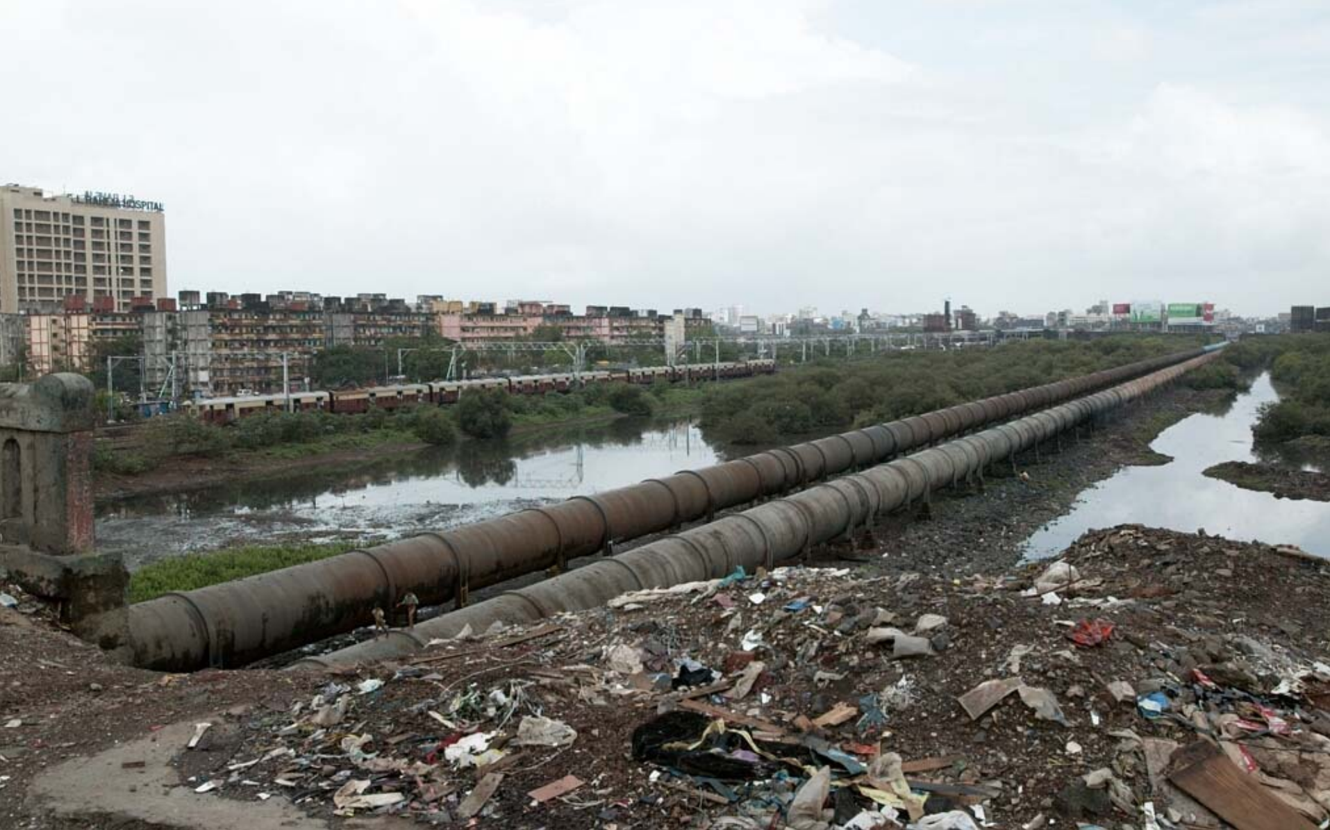
DESTRUCTION OF MANGROVES
