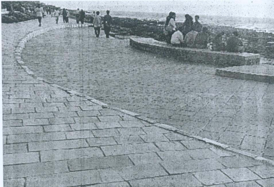
Bandra Bandstand after the redevelopment work
